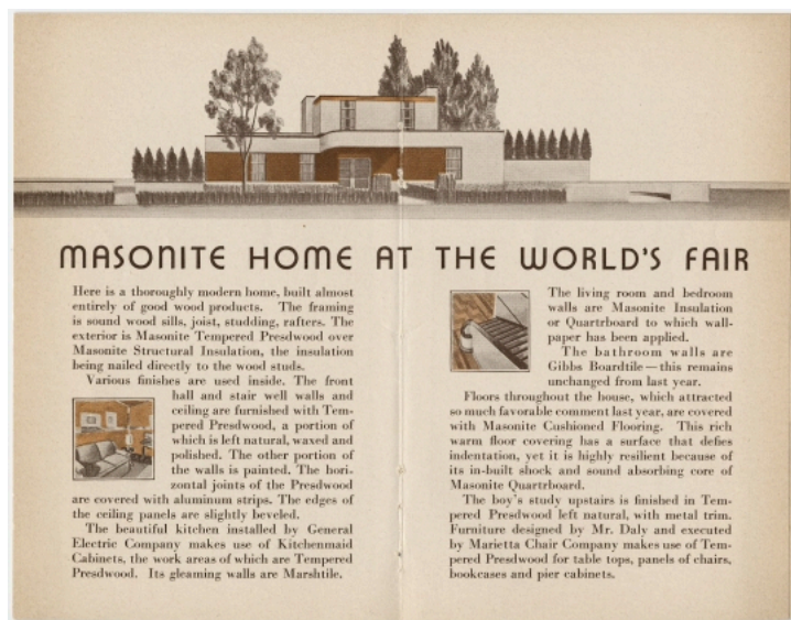
Fig. 4. Masonite House at the Century of Progress International Exposition in Chicago.
