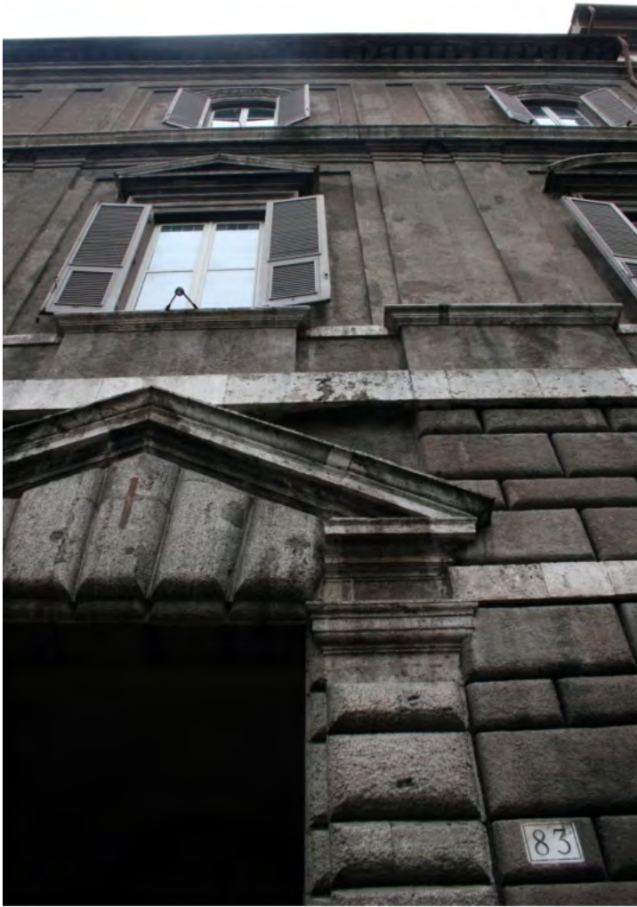
Fig. 5. Palazzo Stati Maccarani, detail showing triple-layering on north façade. Photograph by author.
