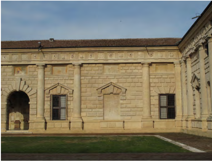
Fig. 57. Palazzo Te, North Courtyard Façade. Photograph by author.
