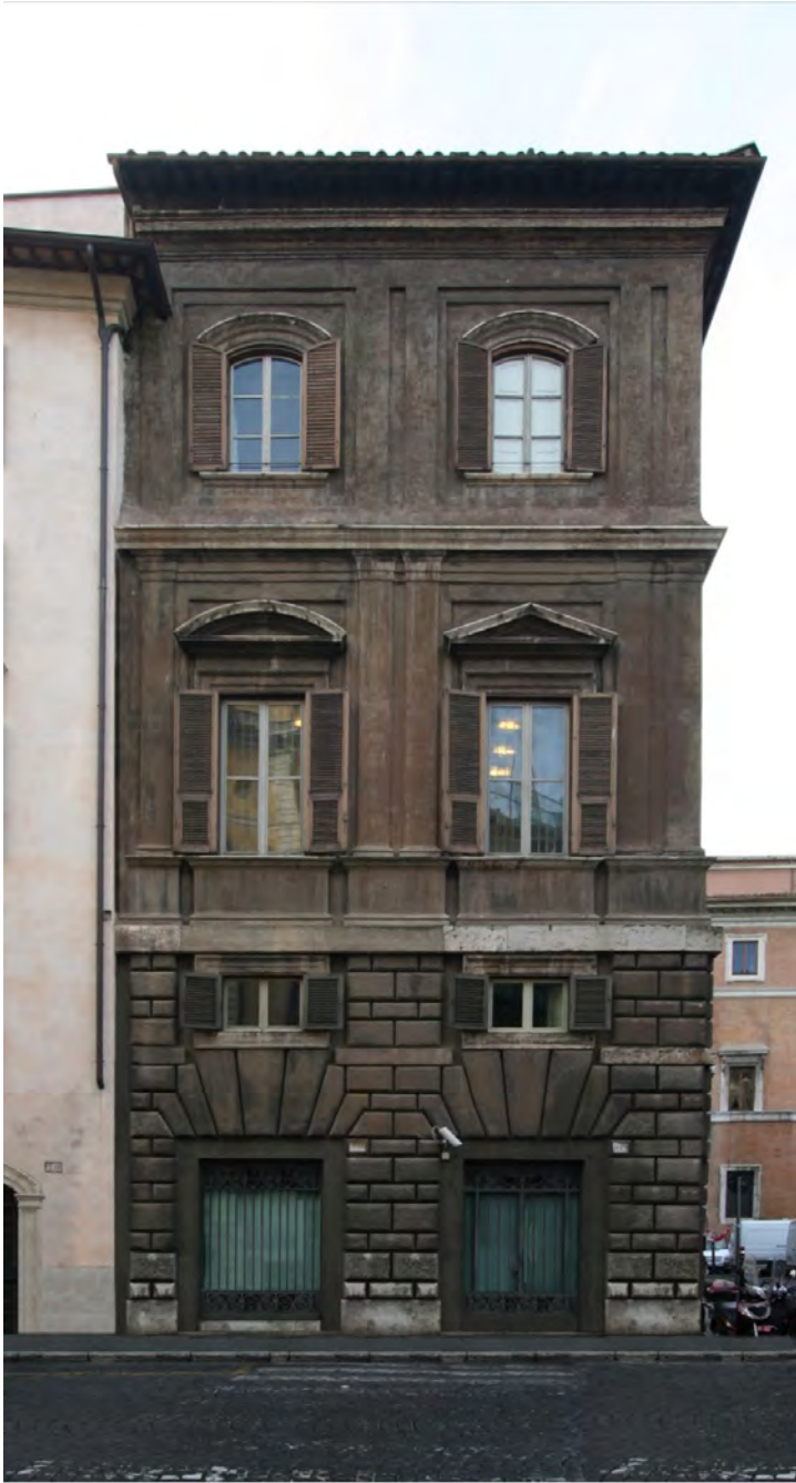
Fig. 59c. Palazzo Stati Maccarani, East Façade. Hypothetical view to indicate how a reveal would maintain the whole module. Representation by author.
