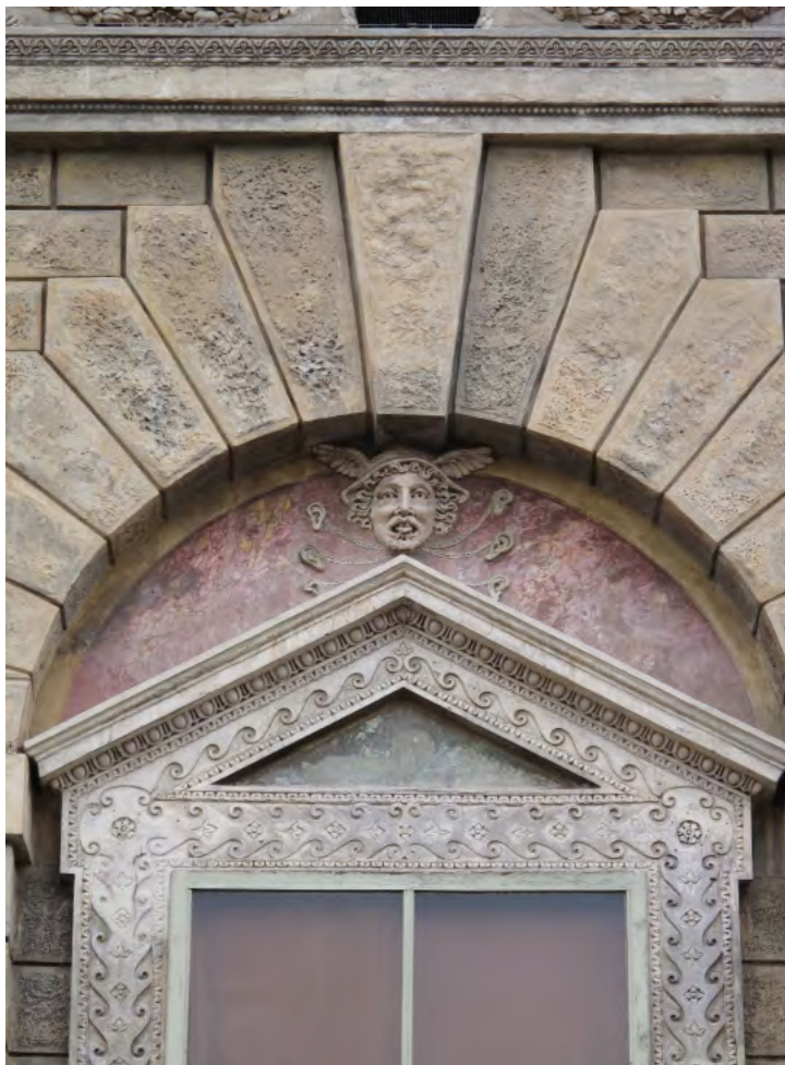
Fig. 31. Giulio Romano's House, Mantua, detail. Photograph by author.
