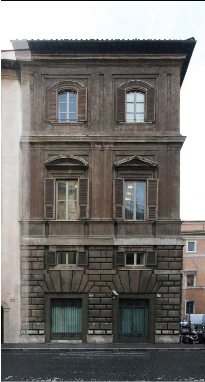
Fig. 59a. Palazzo Stati Maccarani, East Façade. Hypothetical view to indicate extent into adjoining property needed to complete the existing module. Representation by author.
