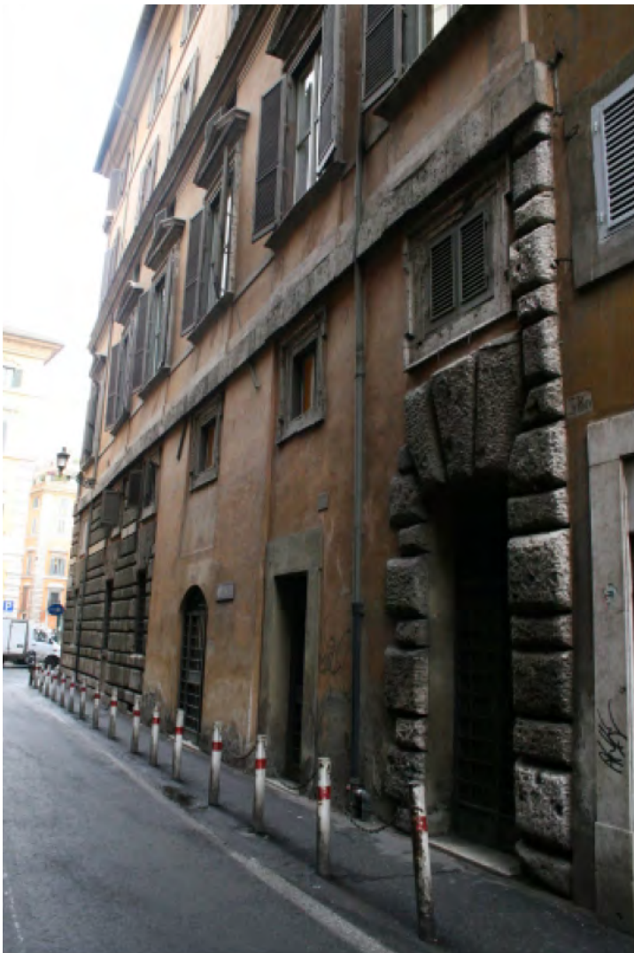
Fig. 1. Giulio Romano, Palazzo Stati Maccarani, Rome, 1522–1524 west façade. Photograph by author.
