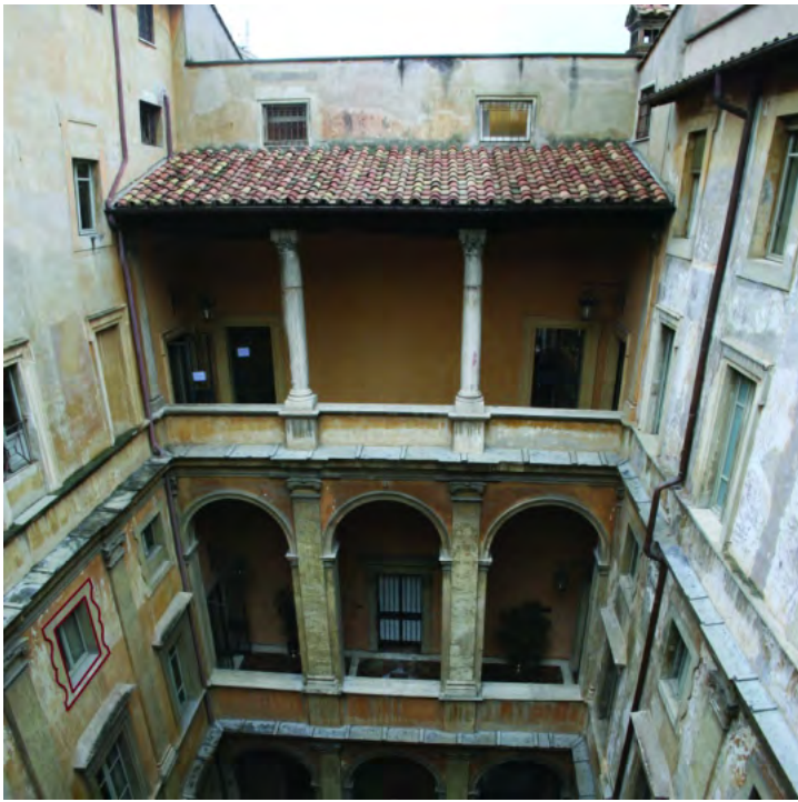
Fig. 51a. Palazzo Stati Maccarani, existing Loggia. Photograph by author.
