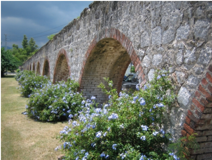
Fig. 15. Hope Aqueduct, near Kingston, Jamaica, ca. 1760s. Photograph by Nicholas Laughlin.
