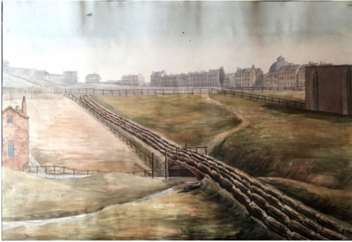
Fig. 1. Soane Office, (drawn by George Basevi), "New River Company, Spa Fields: Wooden Water Pipes," 1814. © Sir John Soane's Museum, London.
