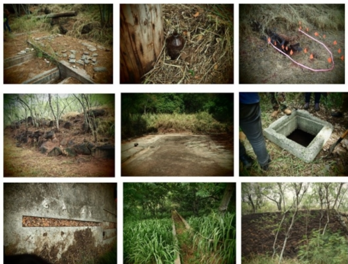
Fig. 5. Extant historical features at Honouliuli National Monument, including concrete compound foundations, drainage catchment structures, retaining walls (low and high), liquor bottles, shell crafts, and ceramics. Photo taken by the author during field school with UH West O’ahu, May–June 2018.
